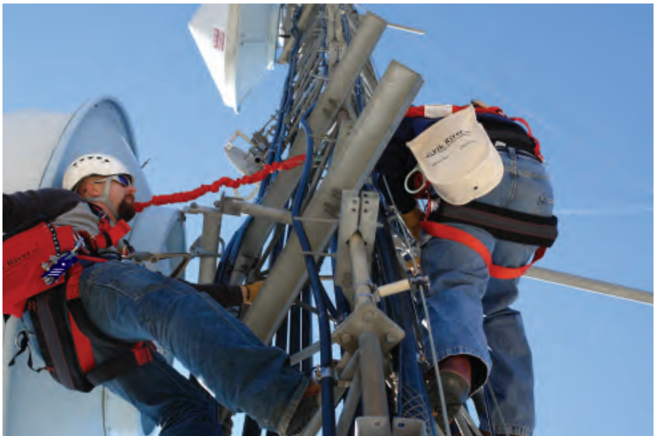
Rebar web positioning assembly being used in a tower climbing application.
